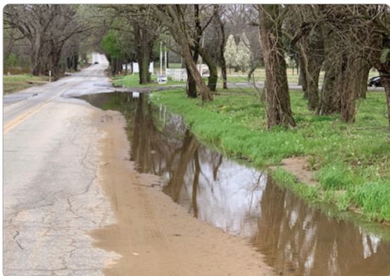
Figure 13. Flooding along W. 81st Street Bike Route
